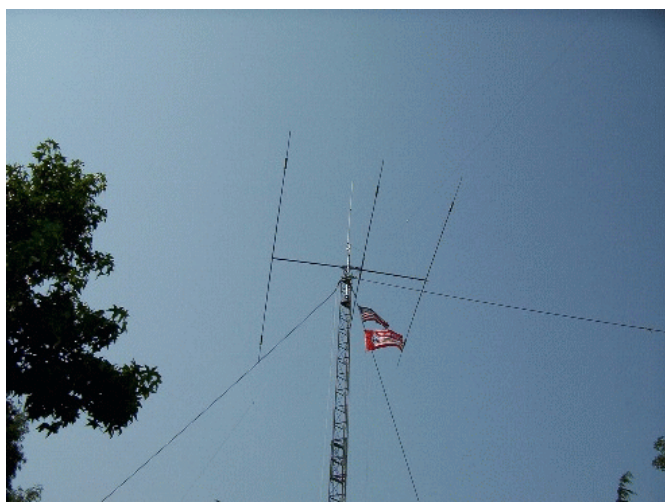
Looking up at the beam antenna from the south, we see our 10-15-20 meter beam, the 2m-1.25m-70cm vertical, and the colors. The tower also supported one end of some HF dipoles, but the wires are not very visible here.
